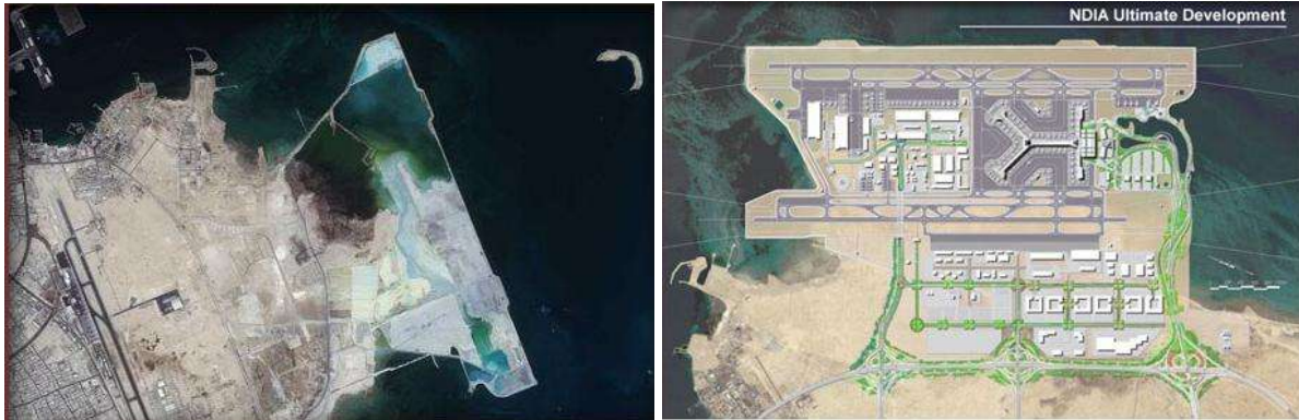
Aerial View of the NDIA construction site and its ultimate development
