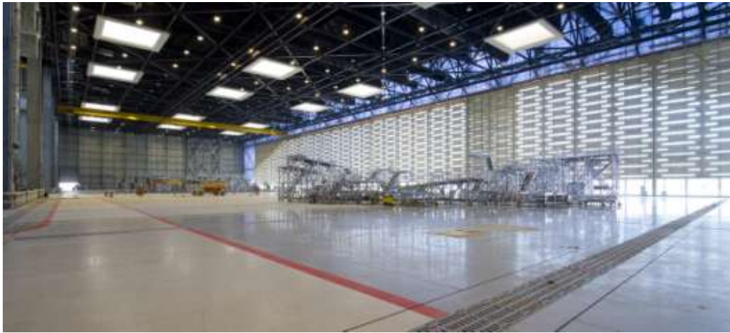
Interior view of the 220m long larger Hangar
